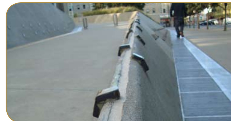
Anti-skate devices, such as metal plates and bolts, disrupt smooth edges and surfaces to deter skateboarding on sidewalks and in other areas
